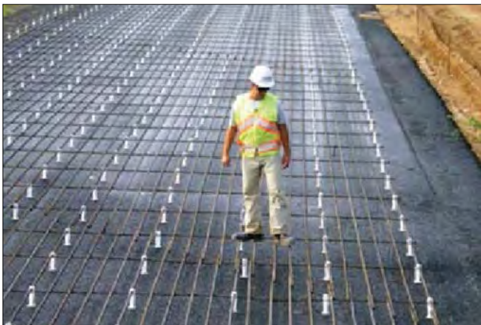
Figure 3. Reinforcement design and placement is critical for good performance.
