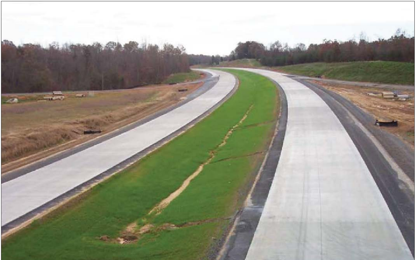
Figure 2. Newly constructed CRCP (Virginia).
