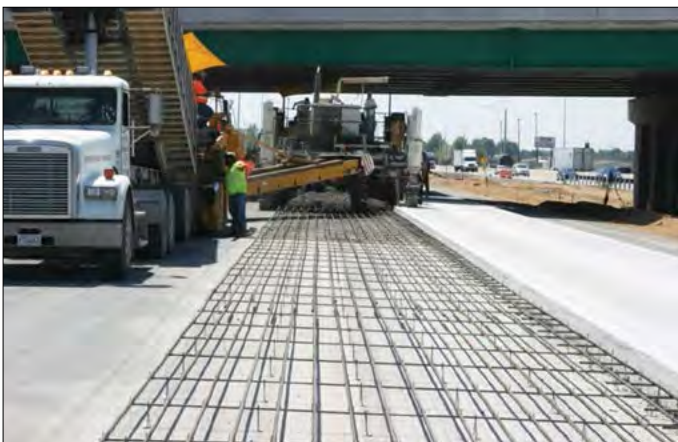
Figure 77. Unbonded CRCP overlay under construction.
