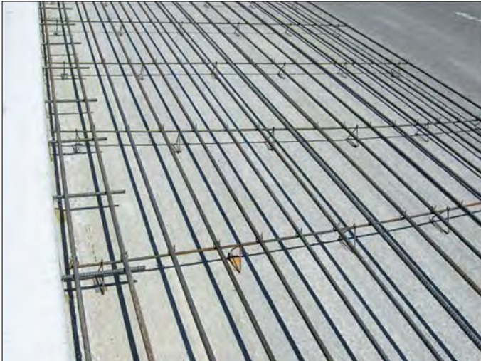
Figure 33. Steel placed on transverse bars assemblies (Illinois).
