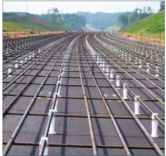
Figure 22. Steel placed on ATB (Virginia).
