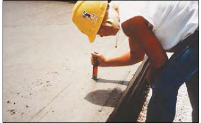
Figure 62. Probing fresh concrete to check the depth of longitudinal steel.
