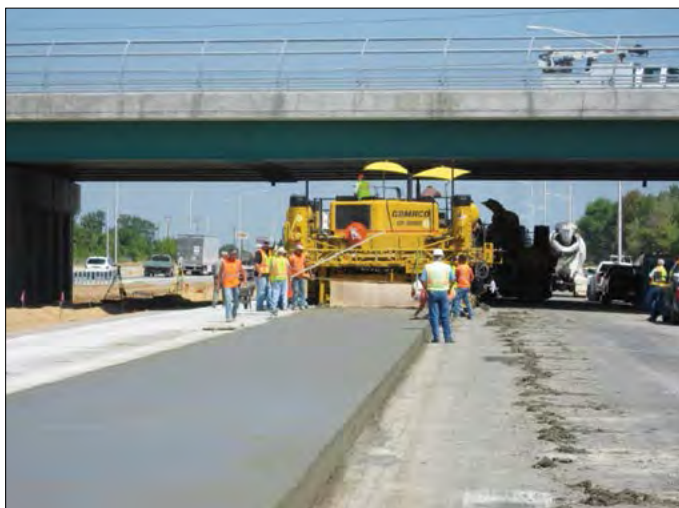
Figure 36. Slip-form paving of CRCP (Illinois).
