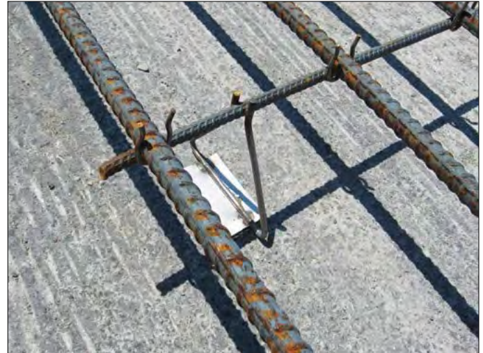
Figure 34. Transverse bar assembly (TBA).
