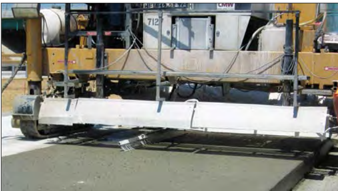
Figure 39. Applying transverse tining on a new CRCP.
