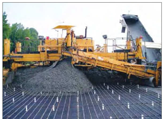
Figure 37. High-speed belt discharge of concrete from end-dump truck (Virginia).
