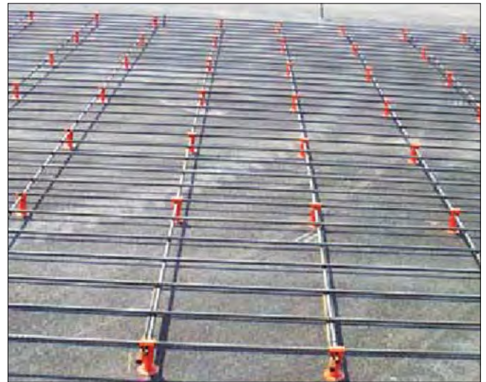
Figure 31. Steel placed on chairs (Texas).
