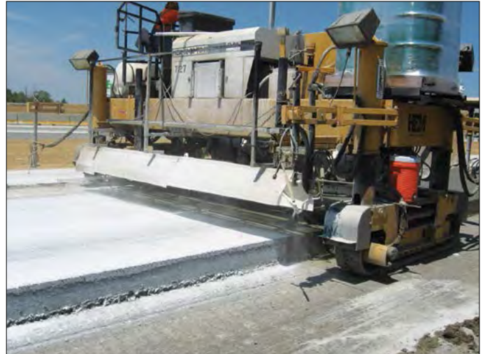
Figure 38. Application of curing compound on slip-formed CRCP.
