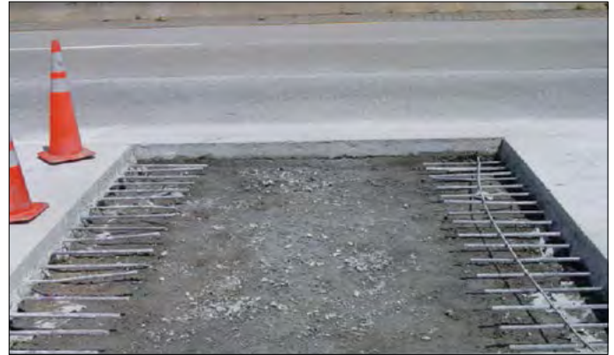
Figure 70. Longitudinal steel exposed in CRCP ready for splicing with new reinforcing steel.
