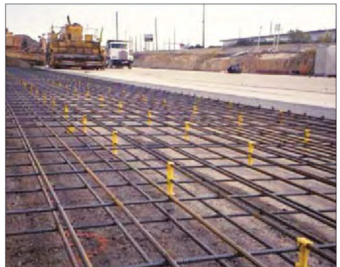
Figure 32. Two layers of steel placed on chairs (Texas).
