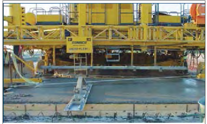
Figure 45. Finishing concrete at end-of-day header.
