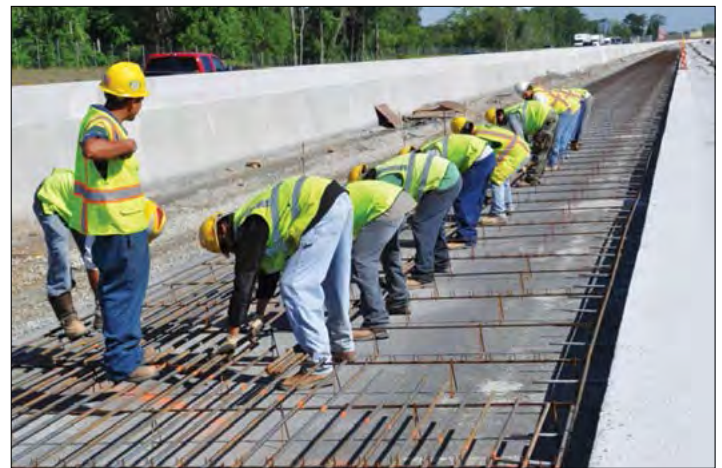
Figure 35. Placing longitudinal steel on TBAs.
