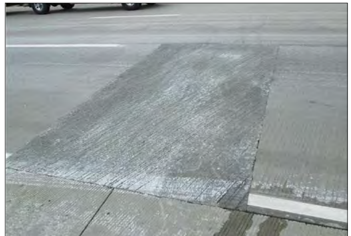
Figure 72. Completed FDR in CRCP.
