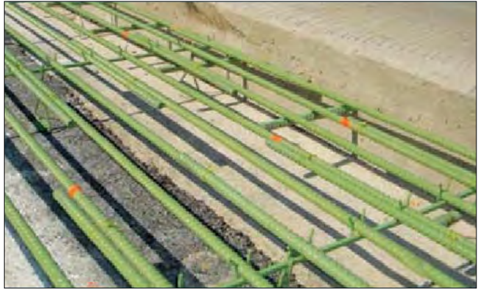
Figure 28. Longitudinal construction joint with tie bars.
