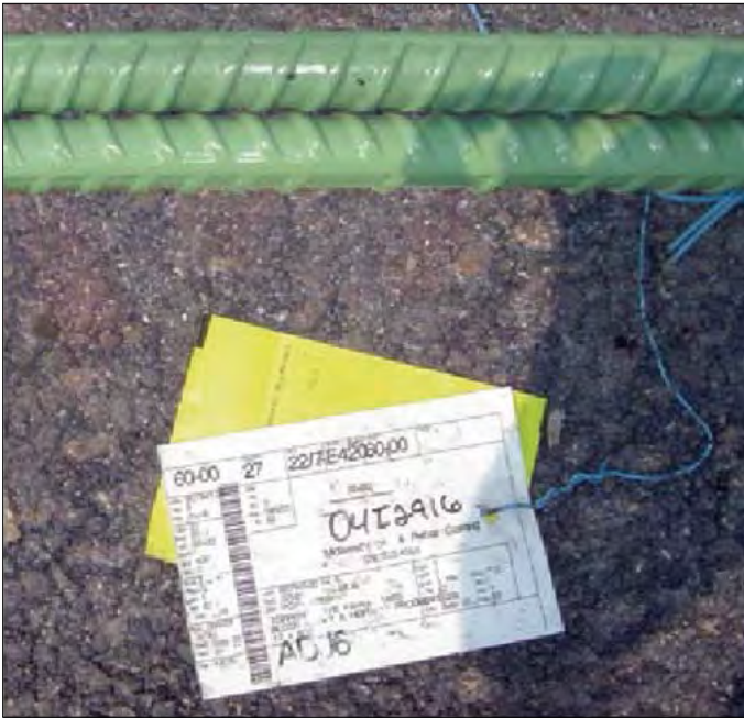
Figure 21. Mill and coating certifications for reinforcing steel.
